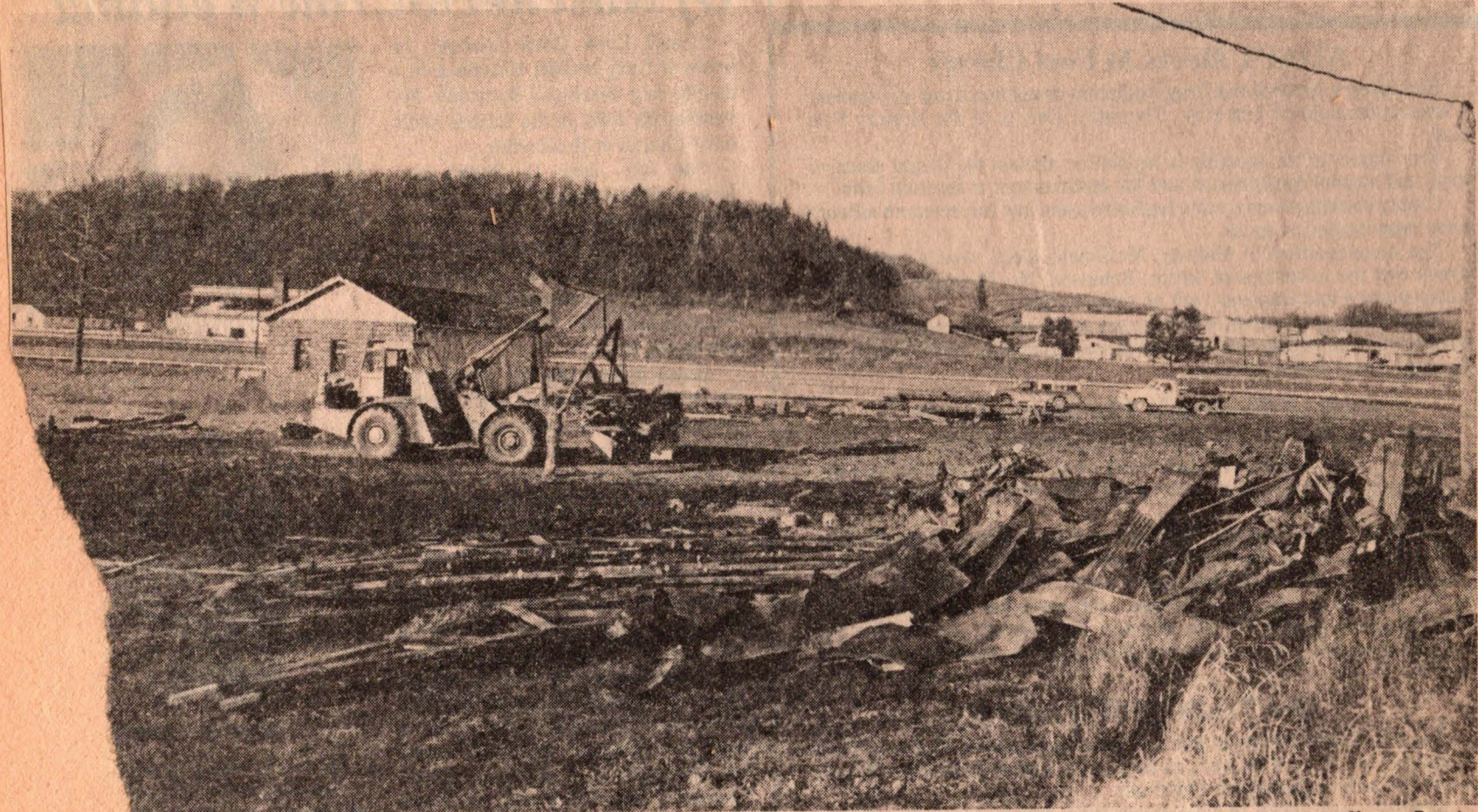
The view of the Washington County Fairgrounds after the razing of the Arden Milling Co.
