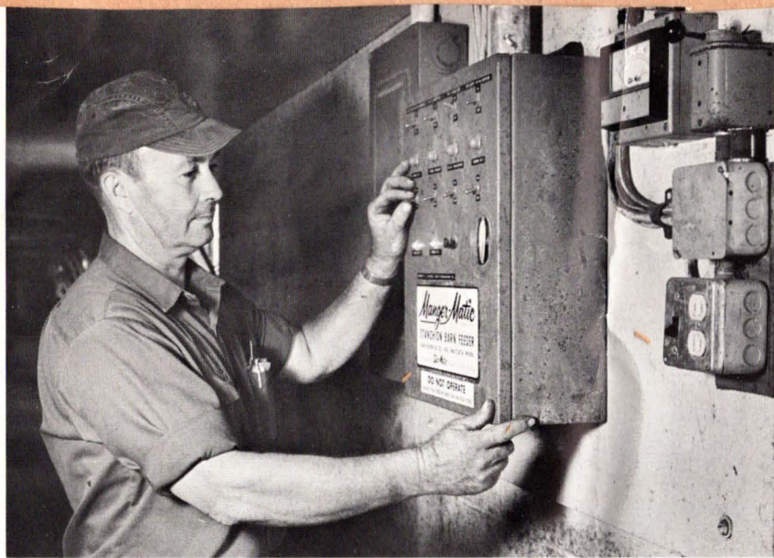
Bob Patton controls the silo unloader, cross conveyor, and his stanchion feed system from this control panel. Two three horsepower motors distribute haylage and corn silage to two rows of feeders in the 36-foot by 150-foot barn.
